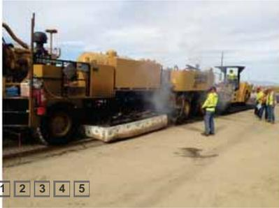
Municipalities and other agencies are taking a closer look at hot in-place recycling (HIR) thanks to a new process by Gallagher Asphalt Corp., located in Thornton, IL. This next step for HIR can recycle 100% of the existing pavement without having to add an overlay, and it can do this for about 30% less cost. The Gallagher Recycled Hot Emulsified Asphalt Treatment — or Re-HEAT — system can also reduce the carbon footprint by 63% compared to a traditional mill-and-fill.
