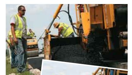
Gallagher Asphalt's road widener paves the first lift of a 6-inch base course of warm mix on Route 53's shoulders
